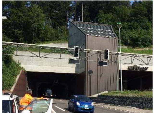
Tunnel Portal Rosenberg
